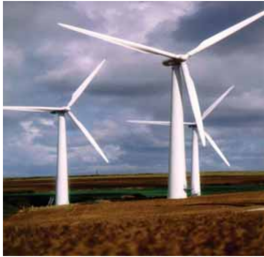
Contracted wind power
