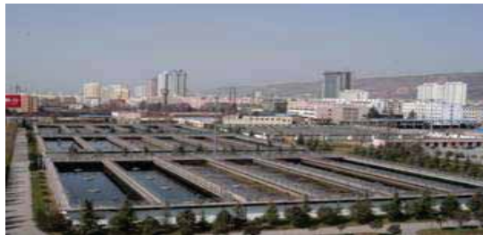
Water distribution/wastewater treatment
